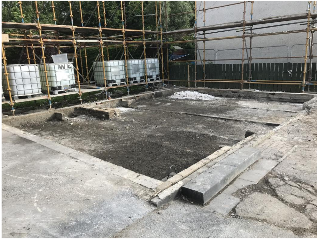
Demolition Complete Retaining Foundations
