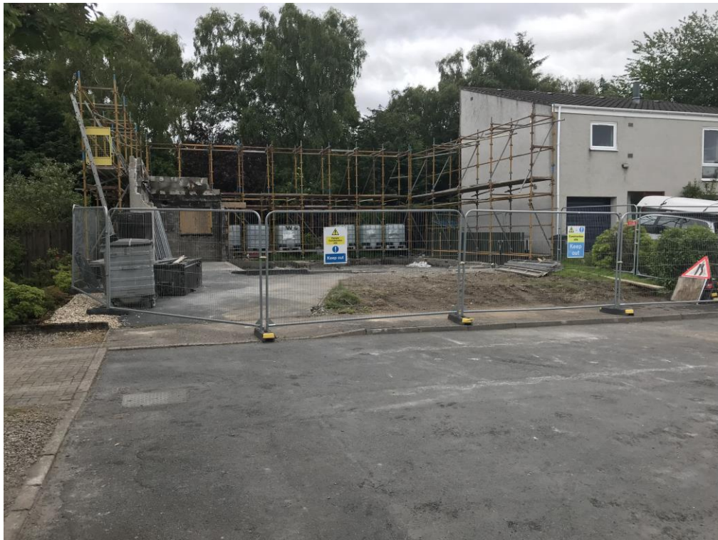
Site Returned to Client for Reconstruction Works to Commence
