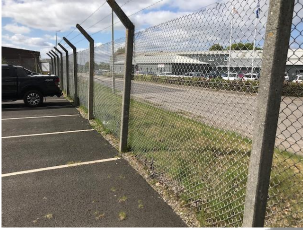
Perimeter Security Fence
