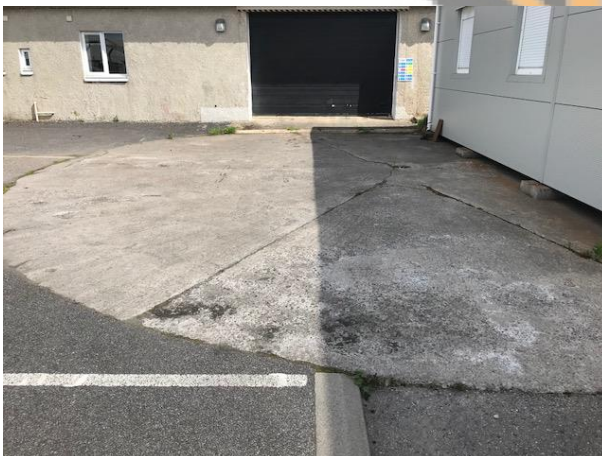
External Hardstanding – Tarmac & Concrete
