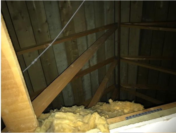
Timber Roof Structure
