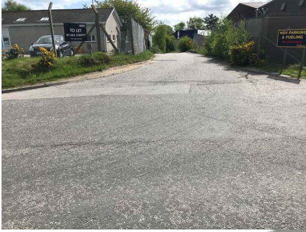
Shared Entrance Road
