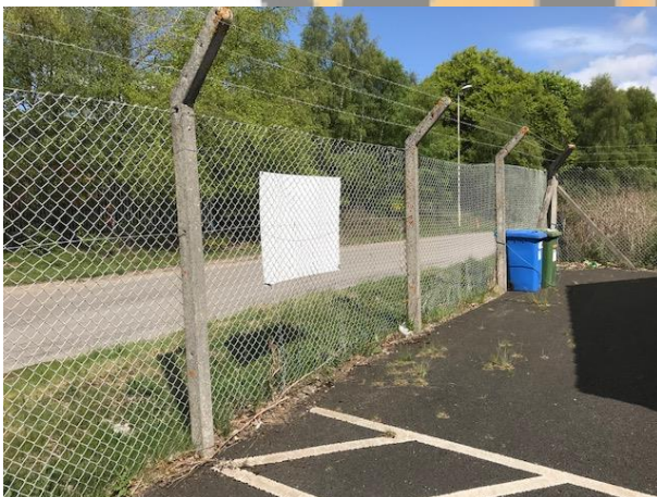
Perimeter Security Fence
