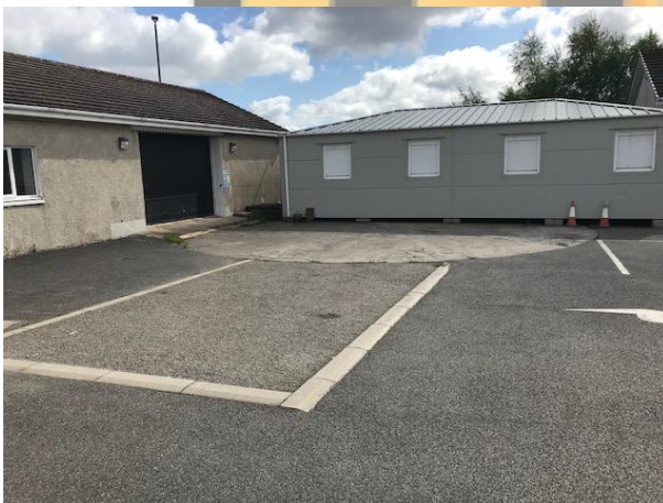
External Hardstanding – Tarmac & Concrete
