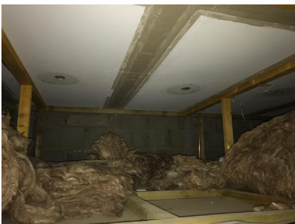
Roof Space – Double Ceiling
